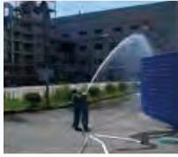
Water Pressure Test
