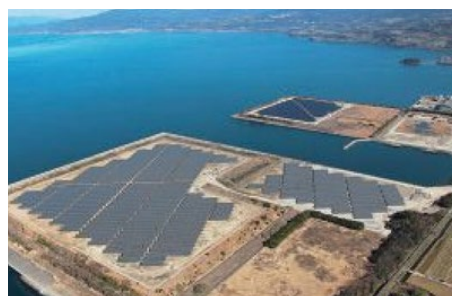
Omura Mega Solar Power Station
