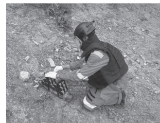
Demolition in progress
