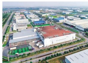
Vietnam Singapore Industrial Park (VSIP) in Hai Phong City, Vietnam
