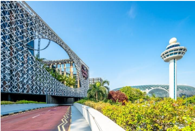
Exterior Façade of Crowne Plaza Changi Airport
