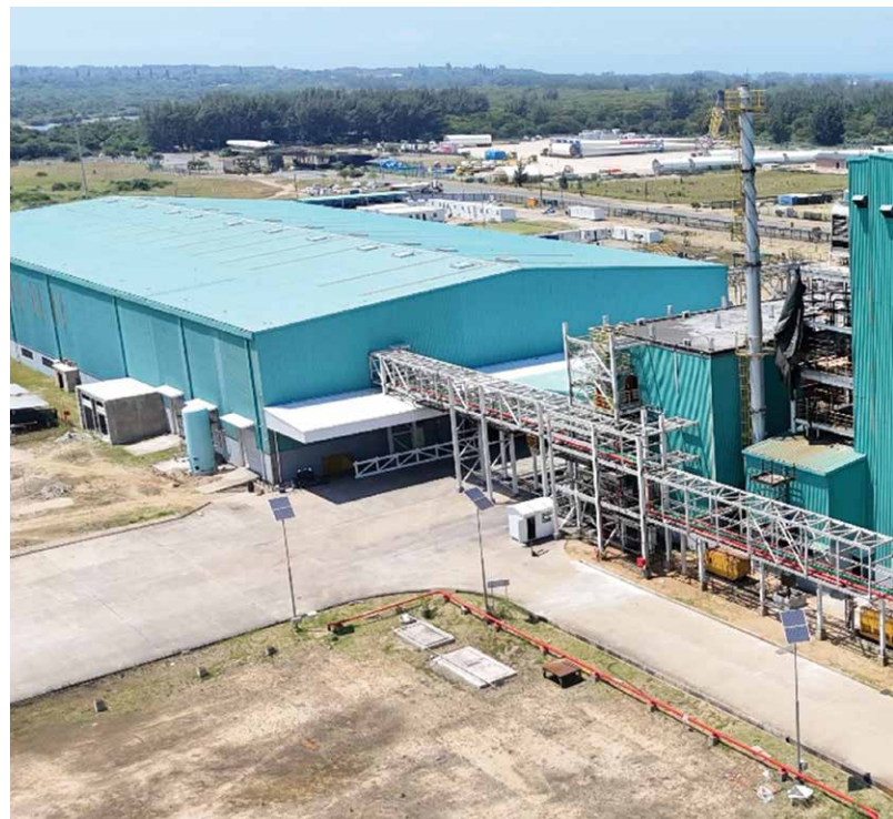
Our new refinery and fractionation plant in South Africa.
