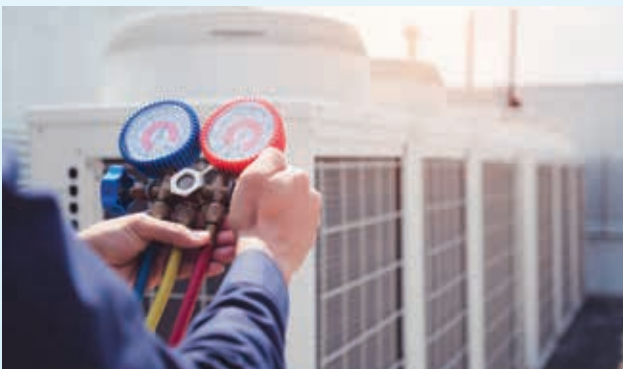
Maintenance in progress (Commercial)
