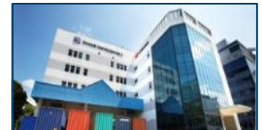
7 Cache Changi DistriCentre 2 3 Changi South Street 3
