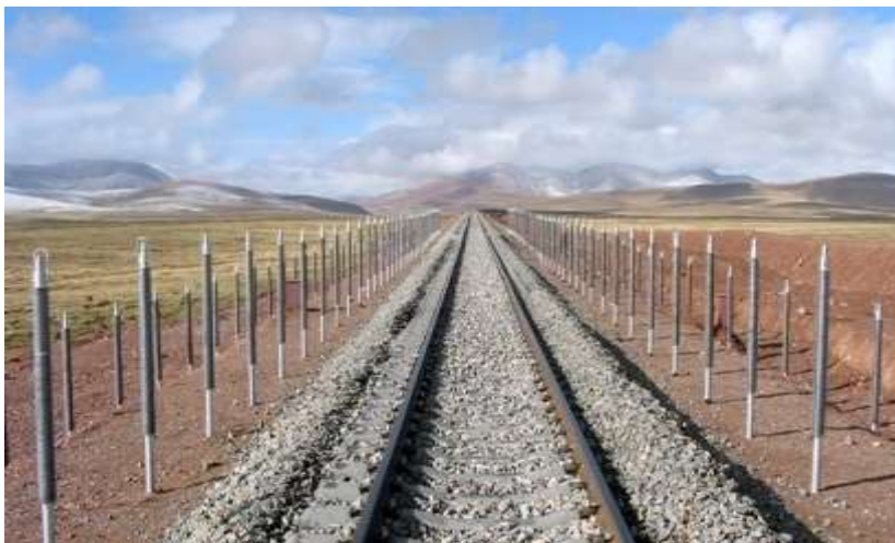
Permafrost treatment technology- heat pipes was adopted in the construction of Qinghai-Tibet Railway
