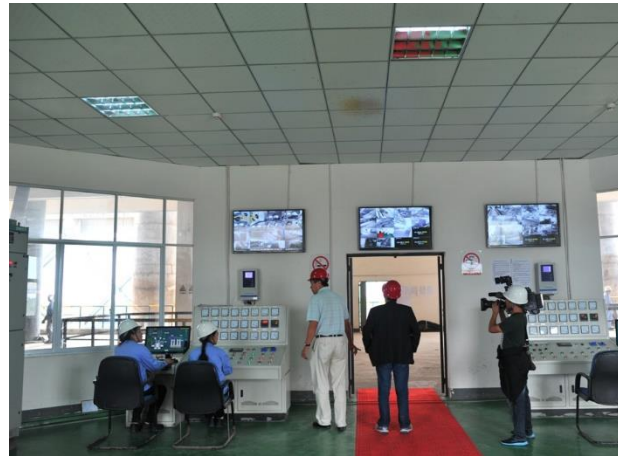
P4 factory control centre
