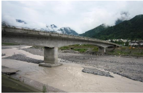
清平场镇大桥 (Qingping Town Bridge)
