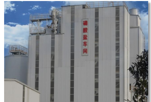
Polyphosphate/ STPP plant
