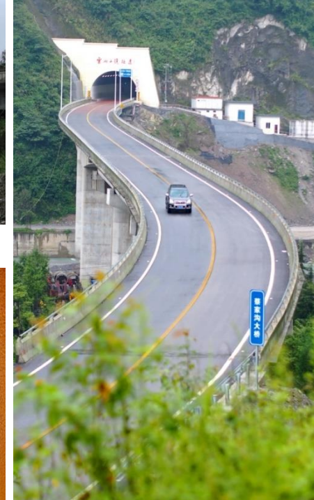
蔡家沟大桥及云湖二号隧道 (Caijiagou Bridge and Yunhu No.2 Tunnel)
