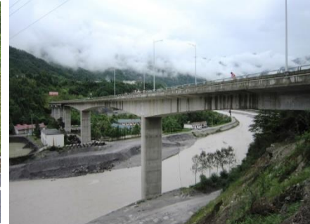
蔡家沟大桥 (Caijiagou Bridge)
