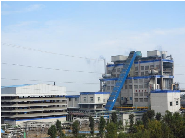
P4 factory / bulk storage
