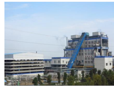
P4 factory / bulk storage
