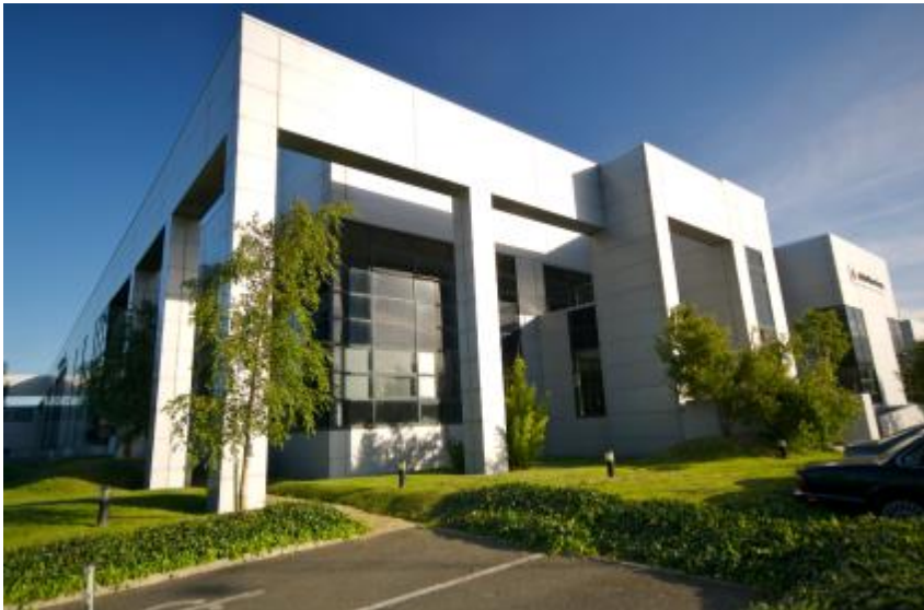
Keppel DC Dublin 1 to undergo upgrading
