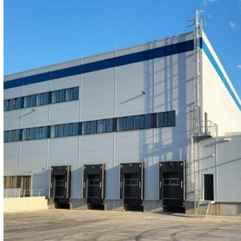
€15 million Lovosice ONE Industrial Park I The Czech Republic
