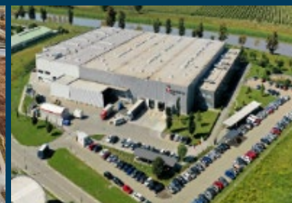
Moravia Industrial Park Uherské Hradiště, The Czech Republic
