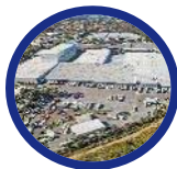
69 Sargents Road, Minchinbury
