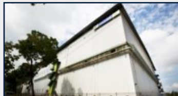
2 ALOG Cold Centre 2 Fishery Port Road
