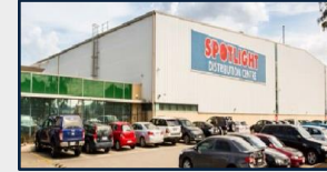
19 217 – 225 Boundary Road, Laverton North
