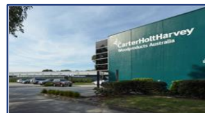
24 41 - 45 Hydrive Close, Dandenong South
