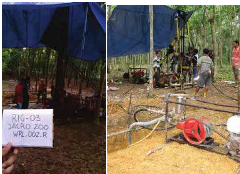
Figure 5:1 WRL Drilling Operations
