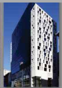
77 King Street Office Tower, Sydney
