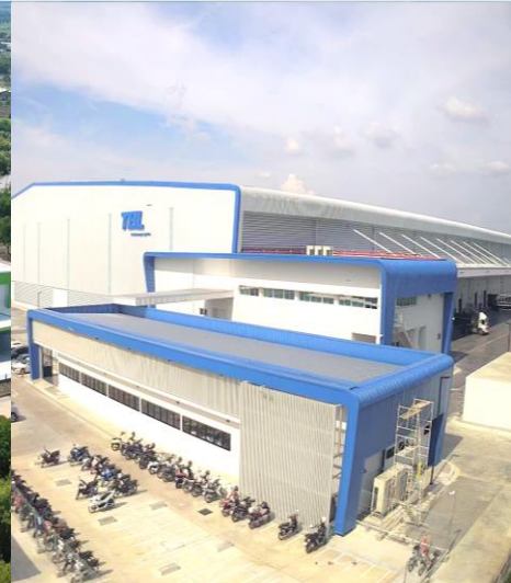
Frasers Property Logistics Park (Wangnoi 2), Ayutthaya
