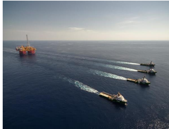
Towage and positioning of the INPEX-operated Ichthys CPF, the world's largest semi-submersible platform
