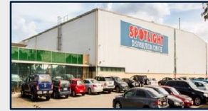
19 217 – 225 Boundary Road, Laverton North
