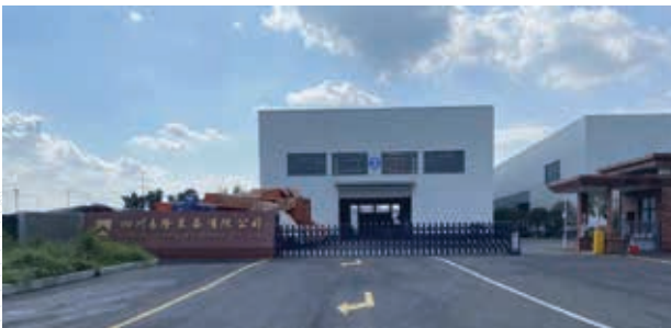
Warehouse at No. 368 Shaqu Industrial Development Zone, Dayi County, Chengdu City, Sichuan Province, PRC. (13,000 square meters)
