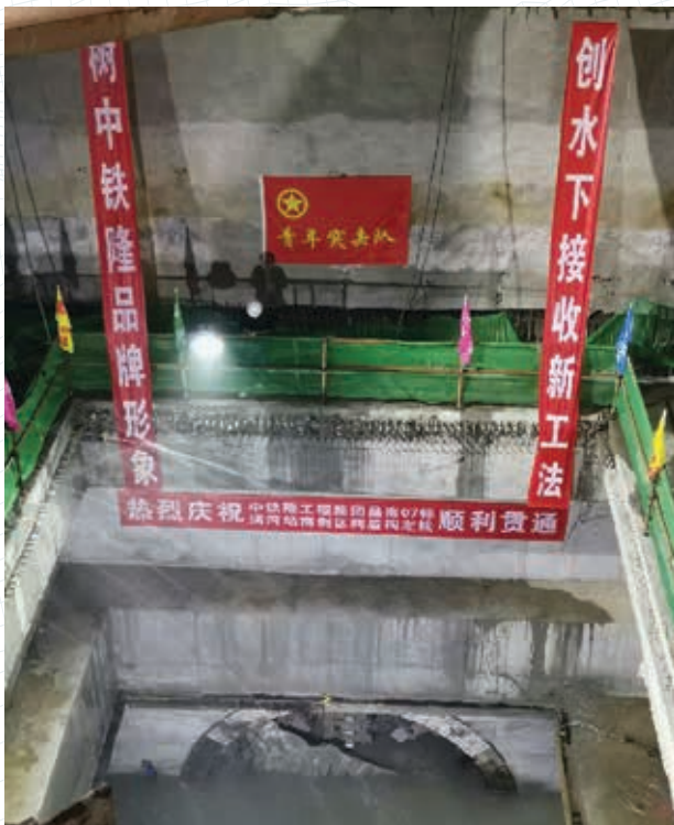
Tunnel boring machine exit through underwater hole in Beijing Metro Changping Line
