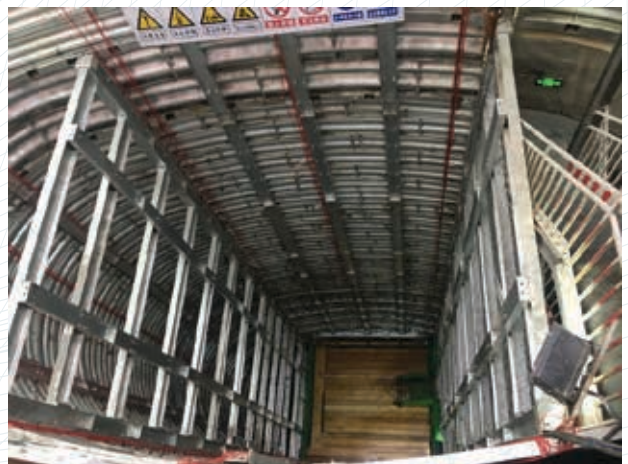
Award winning steel structure used in the Beijing Changping Metro Line
