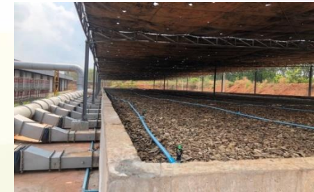
The odor treatment project Bio-filter at Loei factory
