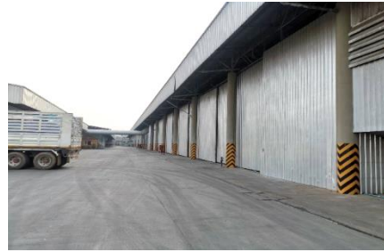
Improved cup lump storage building to closed system at Loei factory
