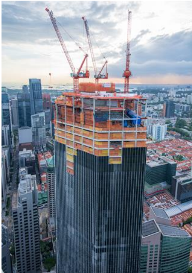
CapitaSpring topping-out at level 51
