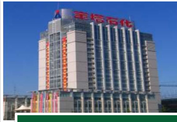
Exterior Board of BTPIC
