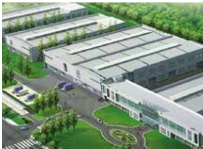
YHI ADVANTI MANUFACTURING (SUZHOU) CO., LTD
