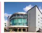
25 Changi South Ave 2
