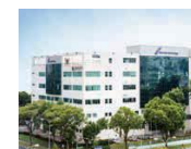
30 Marsiling Industrial Estate Road 8
