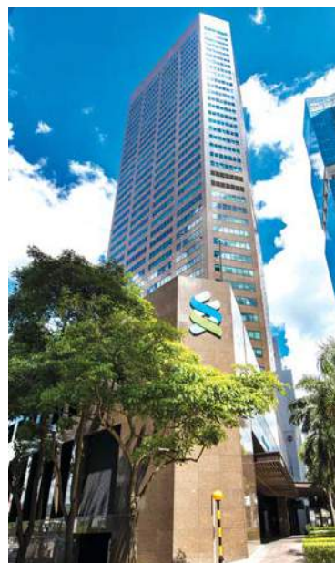
2. Six Battery Road
