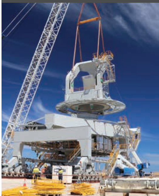
Port Kembla Coal Terminal - Stacker's and Reclaimer
