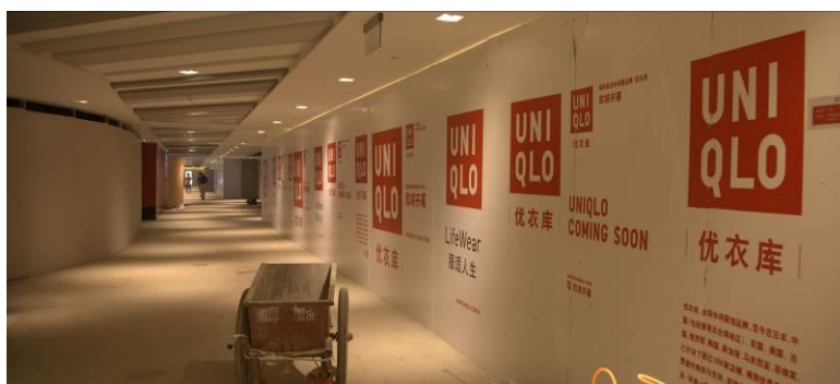
Tenants fit-out work ongoing (ZARA, Massimo Dutti & UNIQLO)
