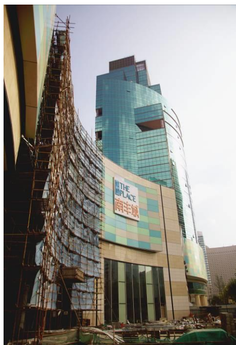
Installation of THE PLACE logo on facade completed
