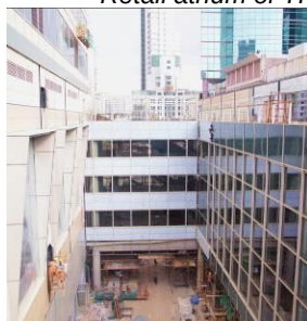
Curtain wall of TP2 link bridge under installation
