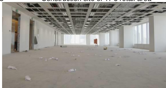
Construction site of TP3 office area
