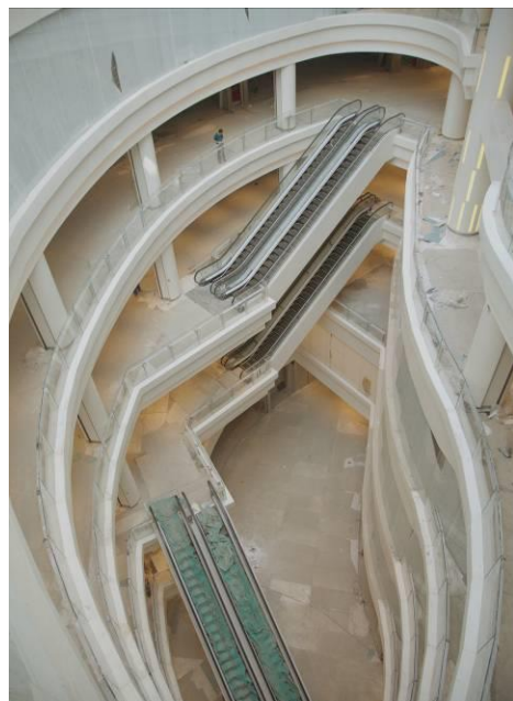
Retail podium of TP3 upon completion of fire service inspection
