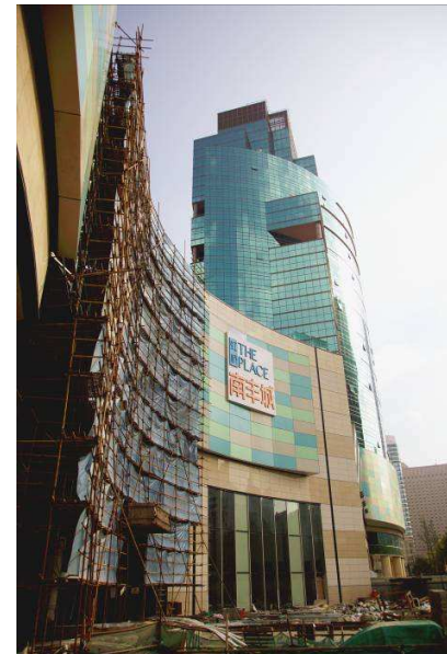
Installation of THE PLACE logo on façade completed
