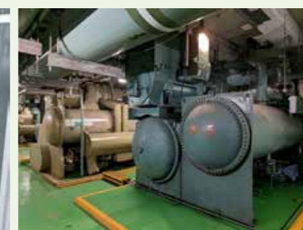
Chiller overhaul and replacement, Festival Walk.
