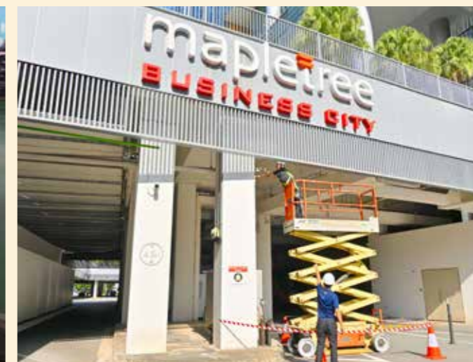
A work-at-height operation underway at MBC.
