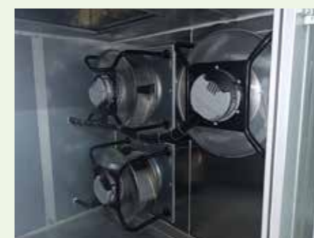
Air-side equipment upgrade with EC Fans, Gateway Plaza.
