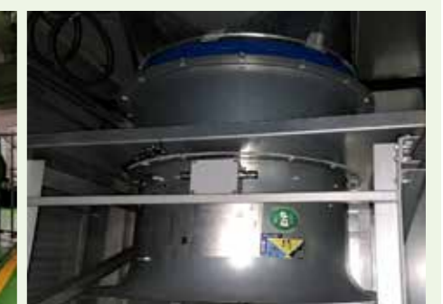
Retrofitting of FCU with EC Fans, VivoCity.
