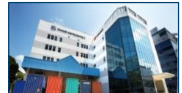
7 Cache Changi DistriCentre 2 3 Changi South Street 3
