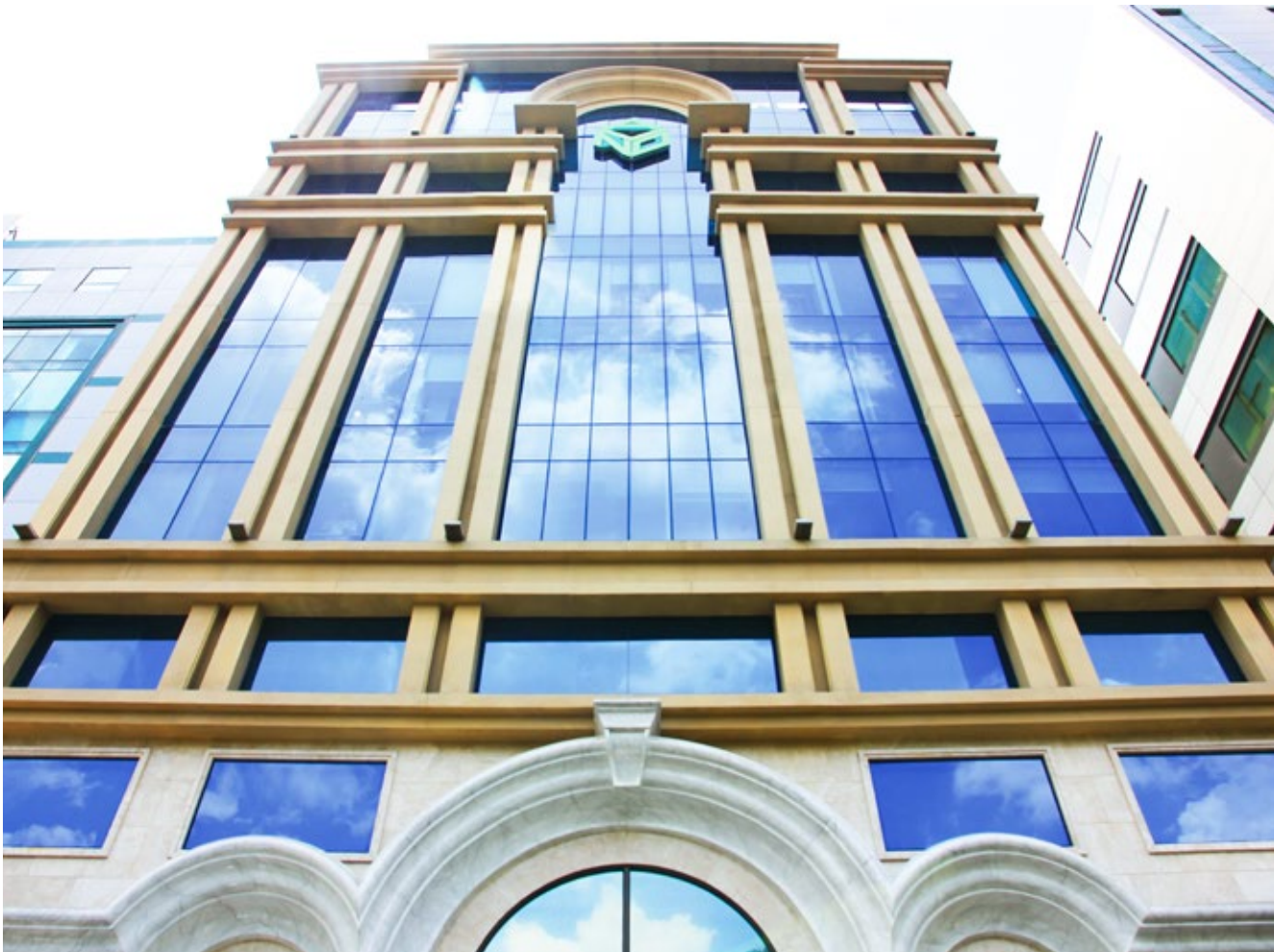
Novaland Office Building (D.1, HCMC)
