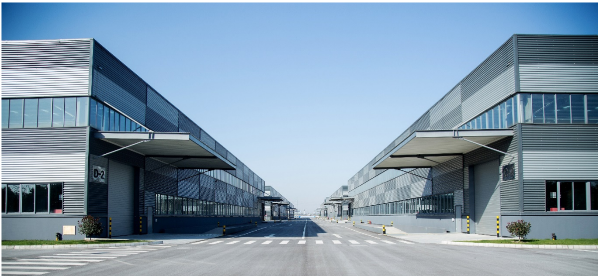
Fervent High Tech Industrial Park Phase 1
