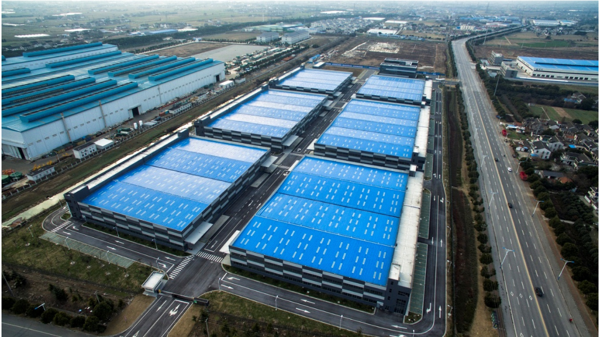
Fervent High Tech Industrial Park Phase 1
