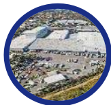
69 Sargents Road, Minchinbury
