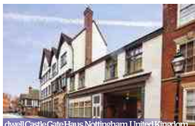
dwell Castle Gate Haus, Nottingham, United Kingdom
