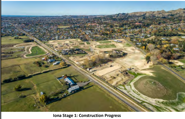
Iona Stage 1: Construction Progress
