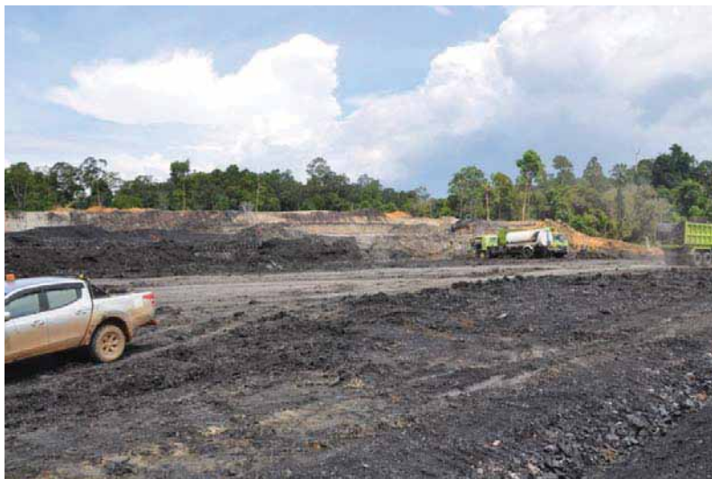
Figure 5:3 Pre-production Operations – BL Block
