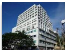
Siloam Hospitals Manado and Hotel Aryaduta Manado
