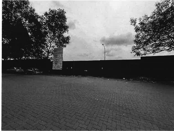
GENERAL VIEW OF THE SUBJECT PROPERTY (TAKEN FROM JALAN ASAM JAWA 16/15)
