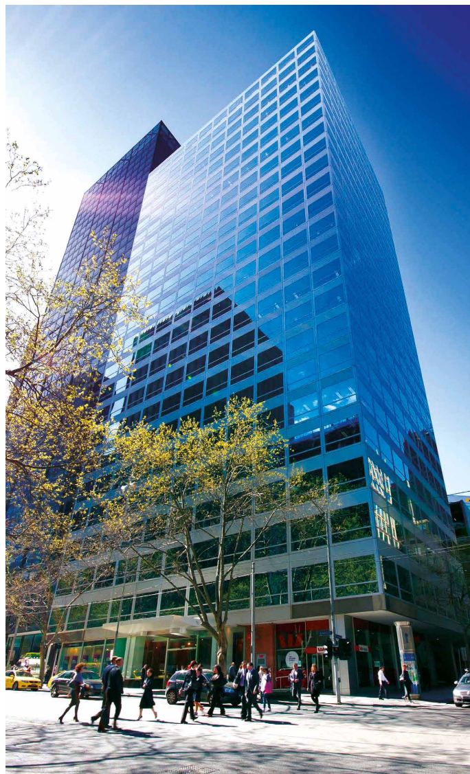
114 William Street, Melbourne, Australia
