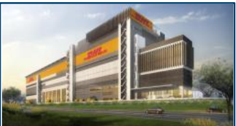
10 DHL Supply Chain ARC 1 Greenwich Drive
