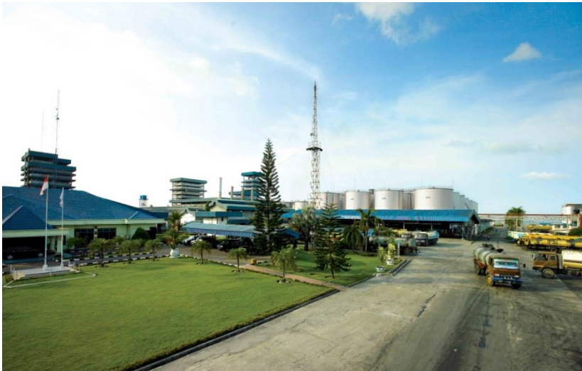
Integrated facility in Sumatra, Indonesia
