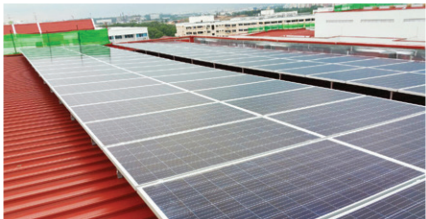
Solar panel installation project on 33 HDB blocks in Tampines.
