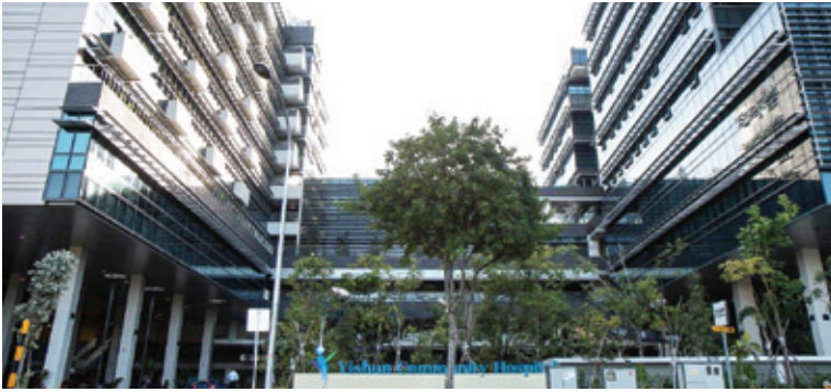
C&P works for Yishun Community Hospital.
