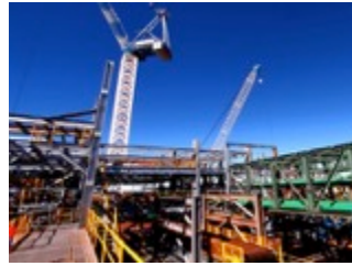
STRUCTURAL MECHANICAL & PIPING INSTALLATION
