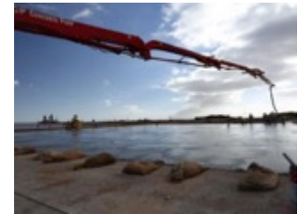
SITE CIVIL WORKS
