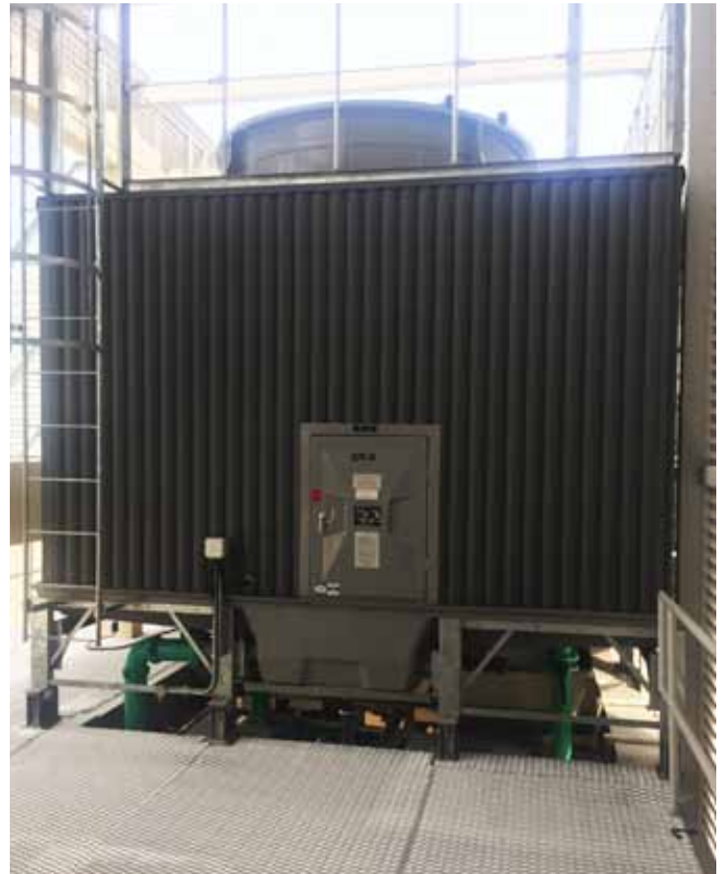
Water consumption in 2017 increased due to the replacement of the hospital's chiller system which is used to cool fluids or dehumidify air in the hospital's facilities.
