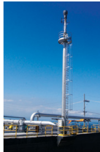
The Renewable Energy Plant at the Cannery, Cagayan de Oro City, Philippines
