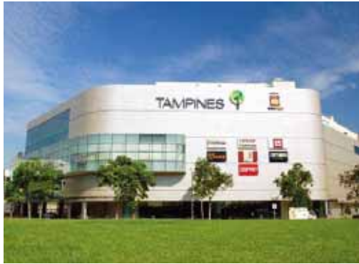
PICTURE 15 – TAMPINES 1, FACADE
