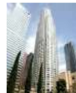
U.S. Bank Tower, Los Angeles (100% stake)
