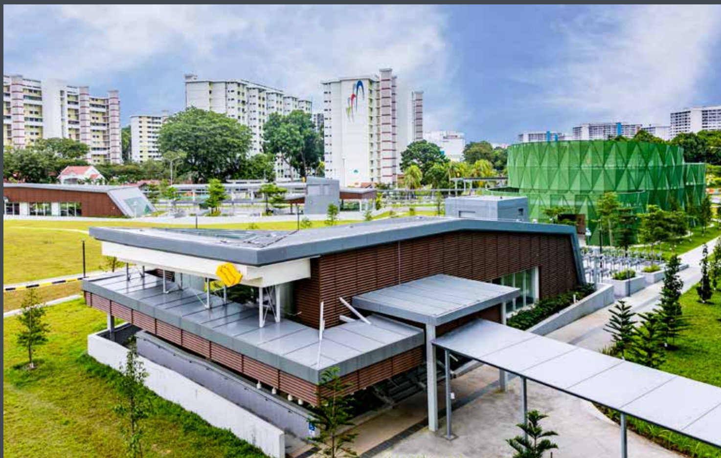
Bedok North MRT station
