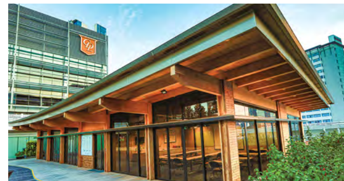
In addition to using sustainably sourced materials certified by Nature’s Barcode™, the SSA features 3,200 square feet of solar PV panels on its roof, generating 60,000 kWh per year to more than fully power the academy.
